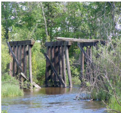
Old Railroad Bridge
